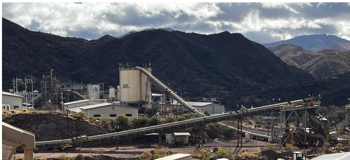
Figure 12-89: General view of the Crushing System
