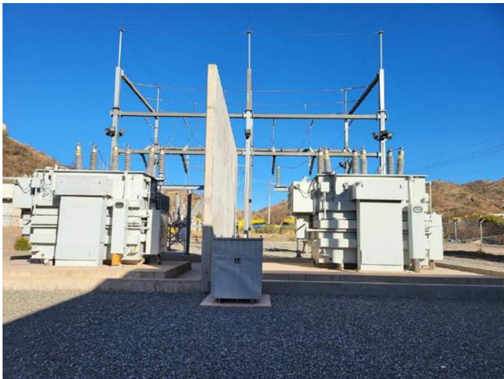
Figure 18-2: Power supply - Step down to 13.2 kVA
