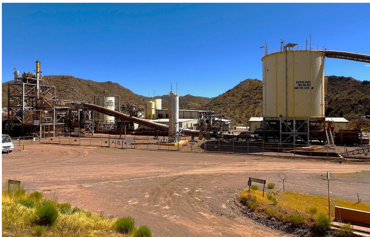
Figure 12-88: General view of the process plant
